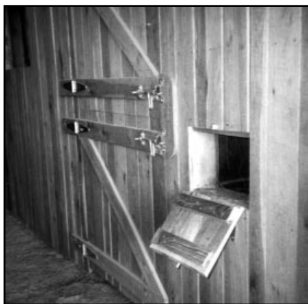
Pictured here is a wheelchair accessible hay feeder that Tom Covington designed.
